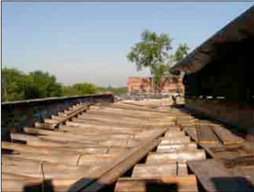
Compressor Room cricket roof shortly before decking was installed.
