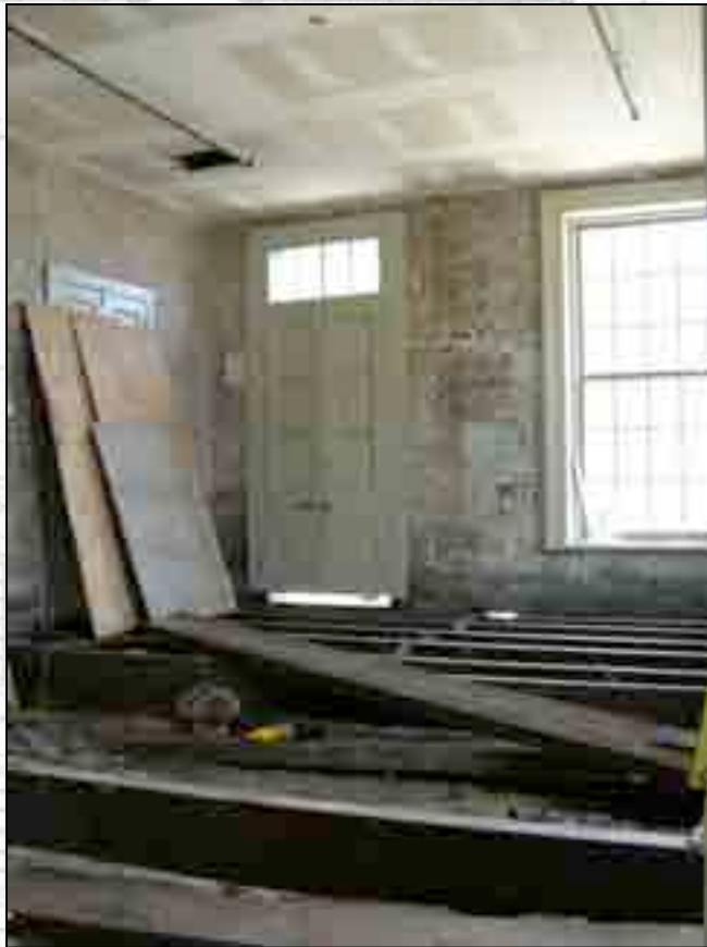
View of southeast room shortly after project began
