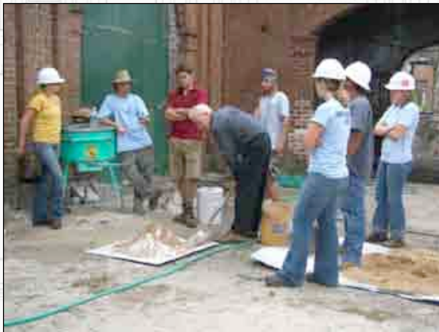
Lynch prepares the mixture of sand and lime for the addition of water.
