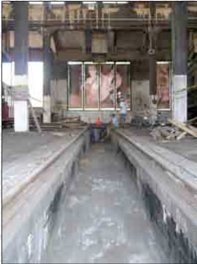
View of lane pit before construction of new pit cover.
