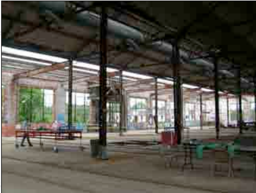
Steel columns during repair work.
