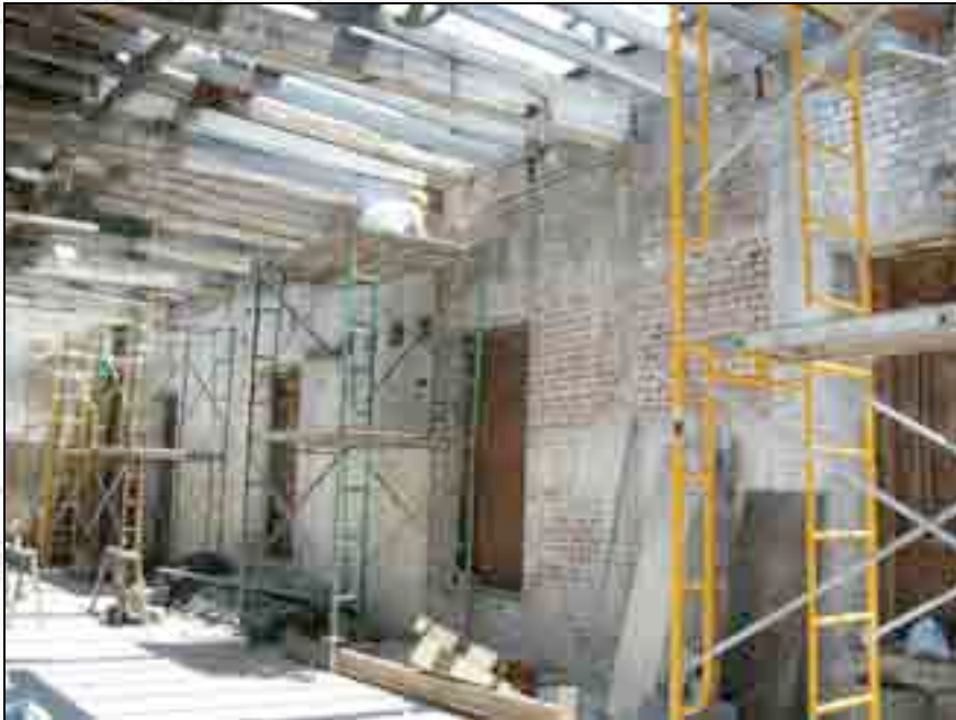
Interior view of the south wall before roof was completed.
