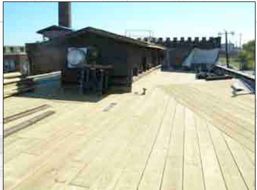
Current view of the roof looking east.
