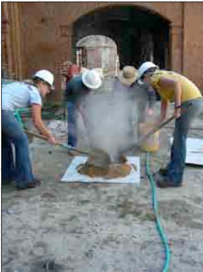
Steam is produced when Lynch and team members mix sand and lime together.
