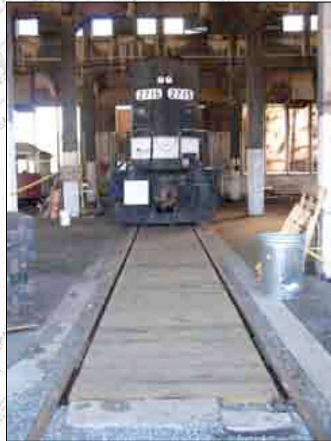
View of pit cover after completion.
