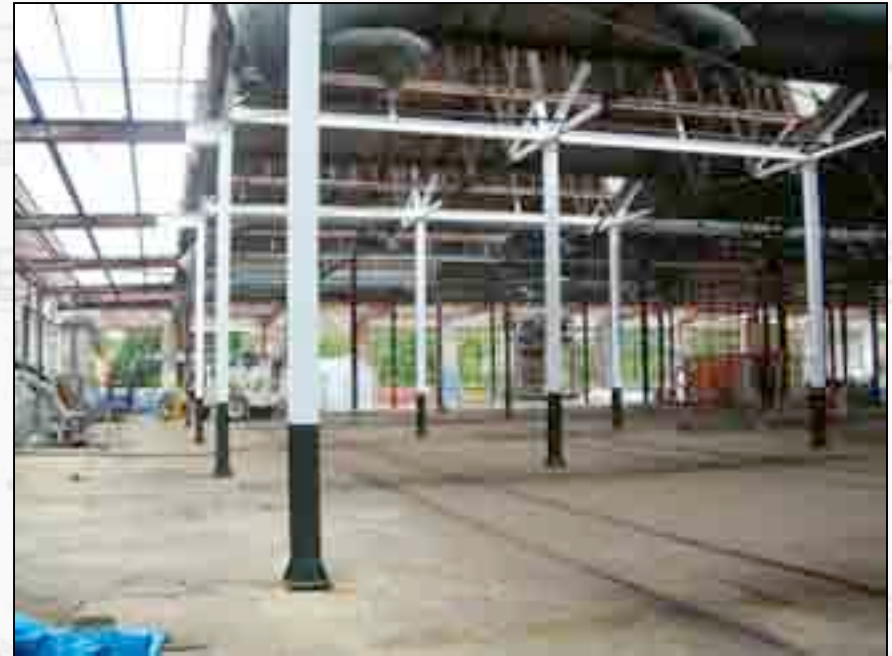
Steel columns after painting.
