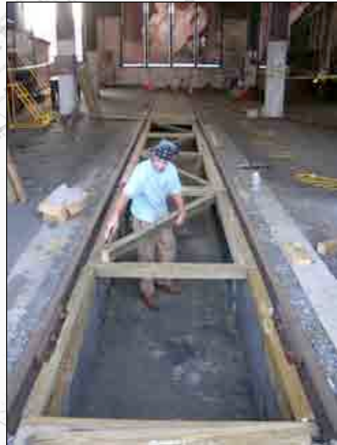
View of pit cover as it is being built.
