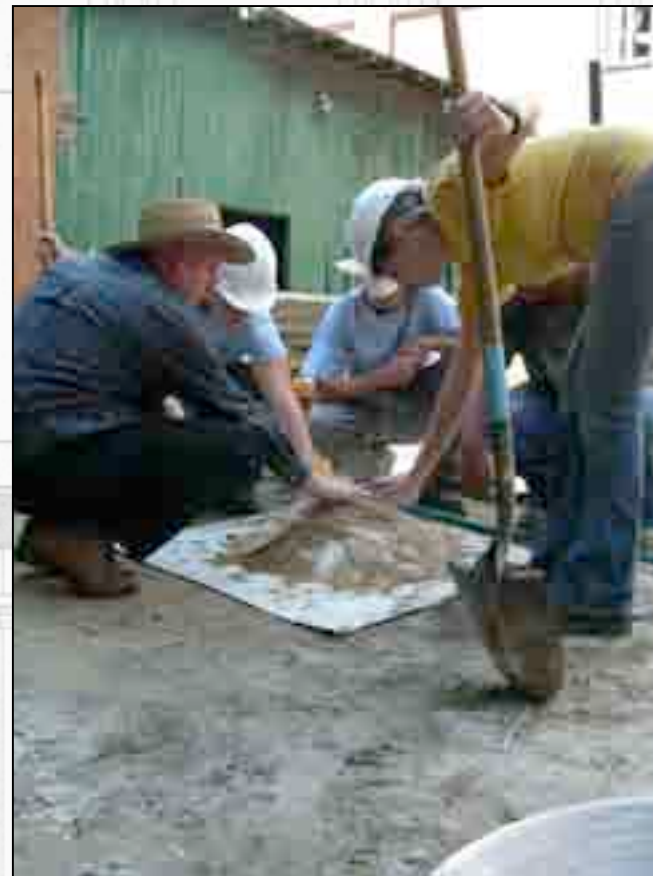
Lynch invites team members to feel the heat coming from the exothermic reaction between the sand and lime.
