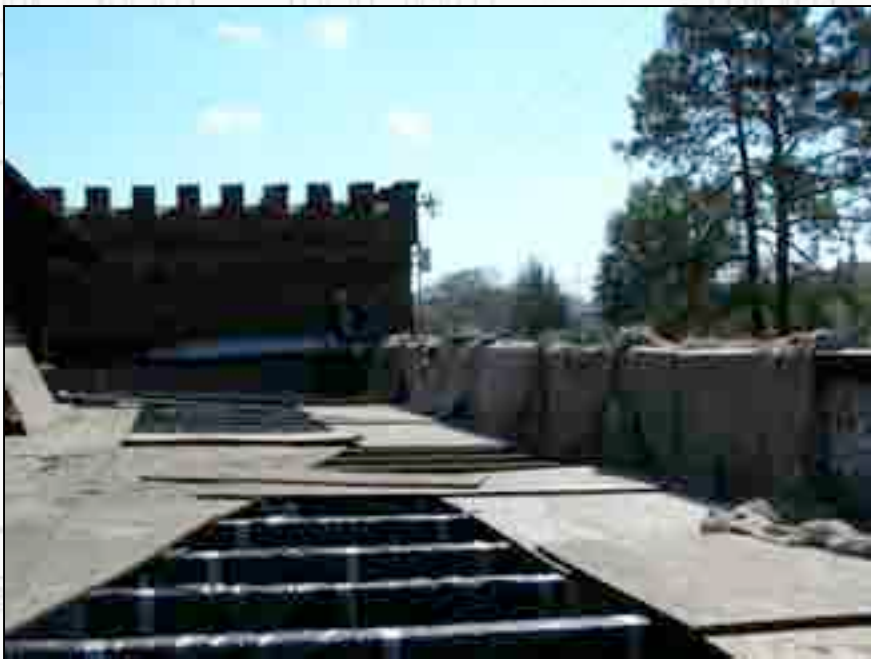
Compressor Room roof shortly after project began.
