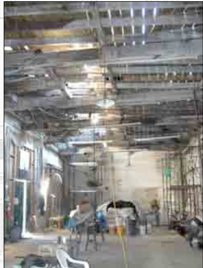
Current interior view.
