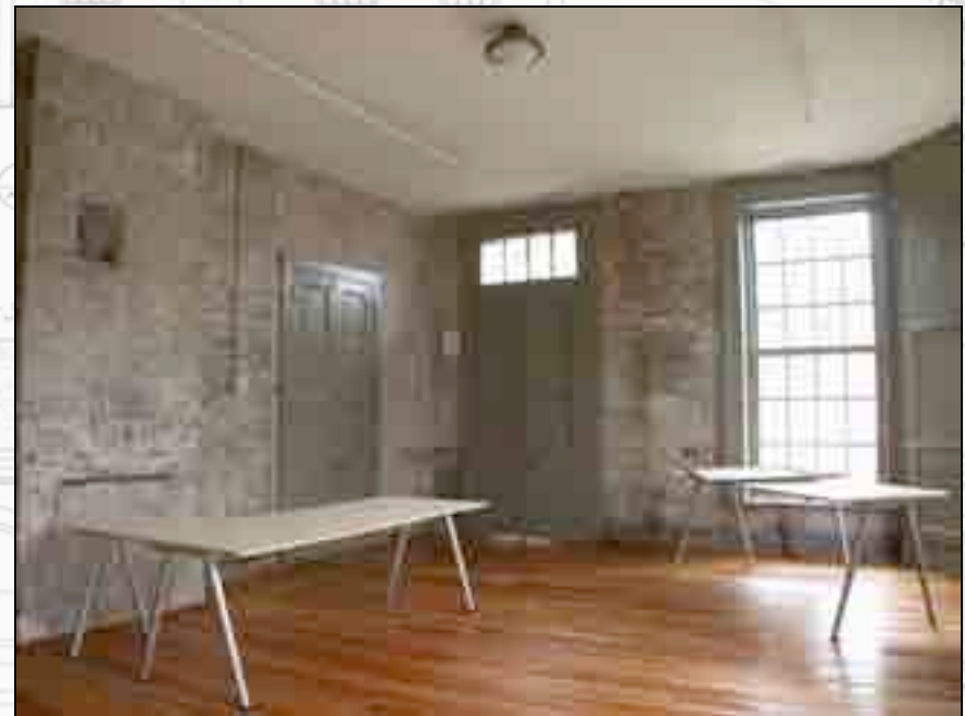
View of room after completion.
