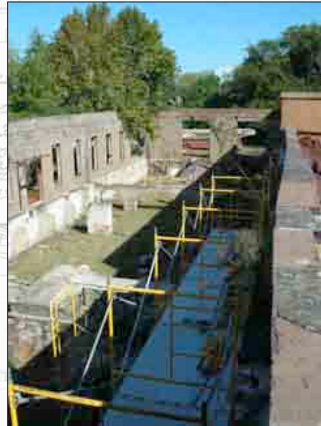
Current aerial view with scaffolding set up for fifth phase of repointing on the east wall.
