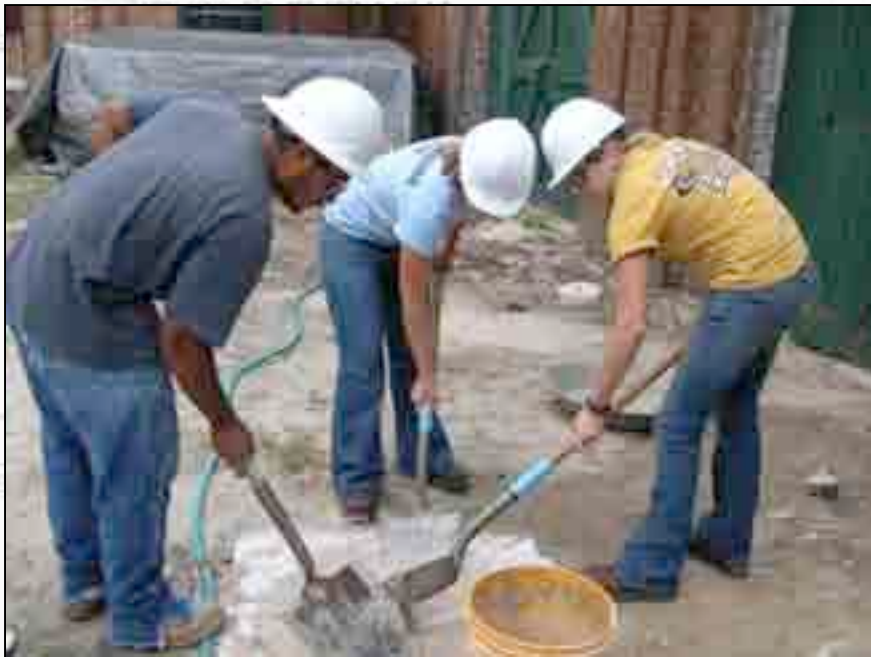
Preservation team members mix lime, sand, and water to make mortar.
