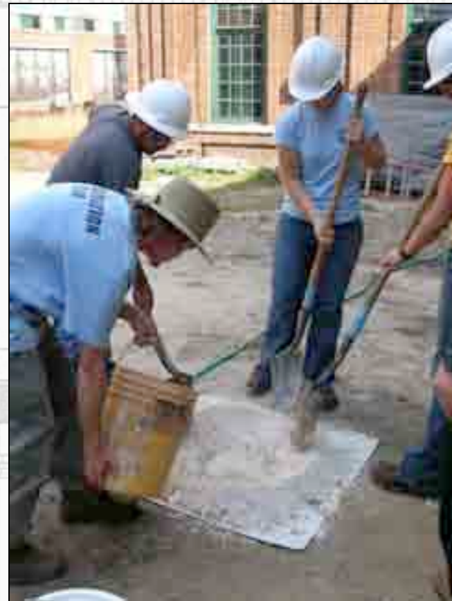
Travis Brown pours water into the mixture while team members stir.
