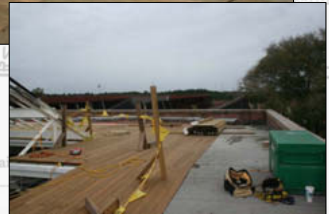
View looking towards the Paint Shop sawtooth roof.
