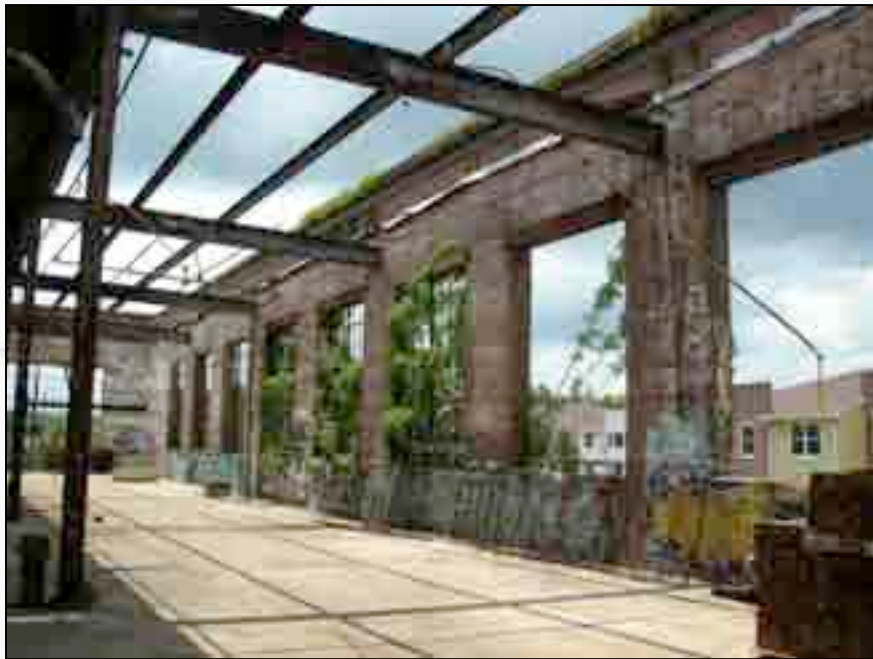
View looking west before all windows were removed.
