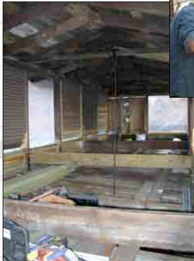
Interior view of the monitor. The wood louvers are being repaired.
