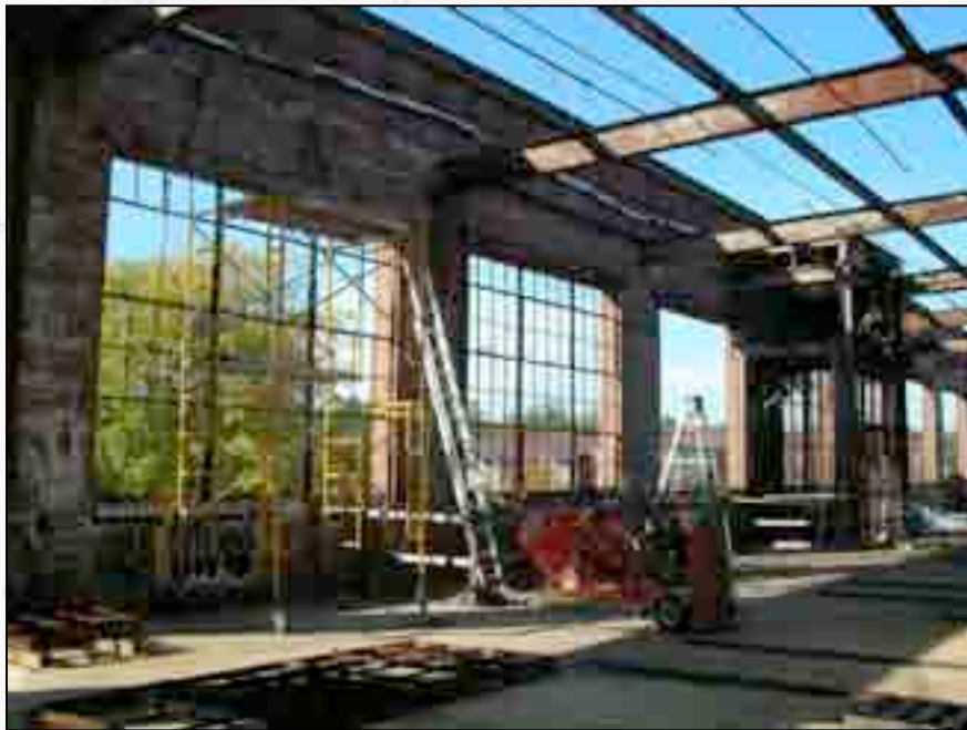
View looking south inside the Paint Shop before windows were removed.
