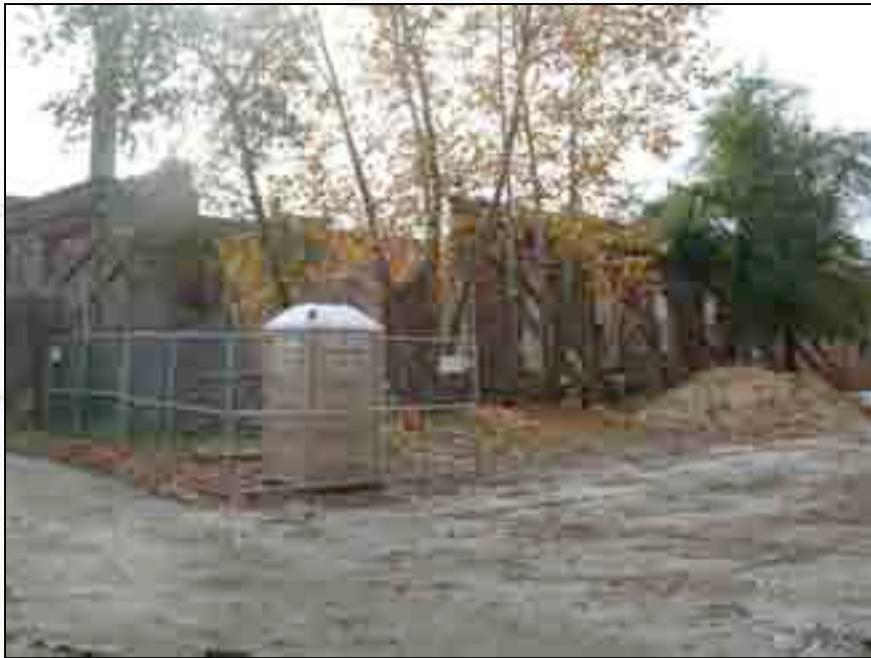
Northwest corner of the Carpentry Shop before tree removal
