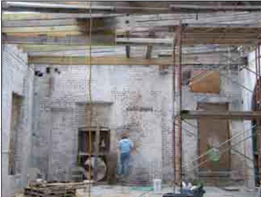
Interior before roof was completed.
