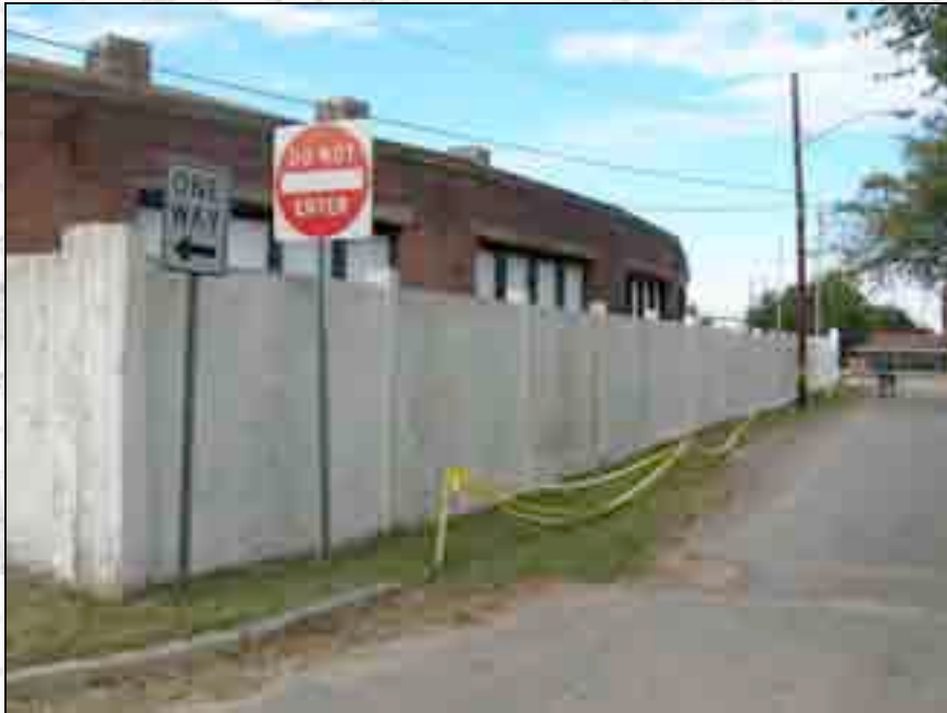
Retaining wall before whitewash application
