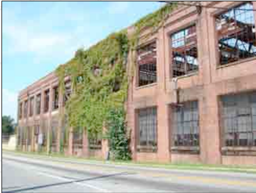
View of west façade before windows were removed.
