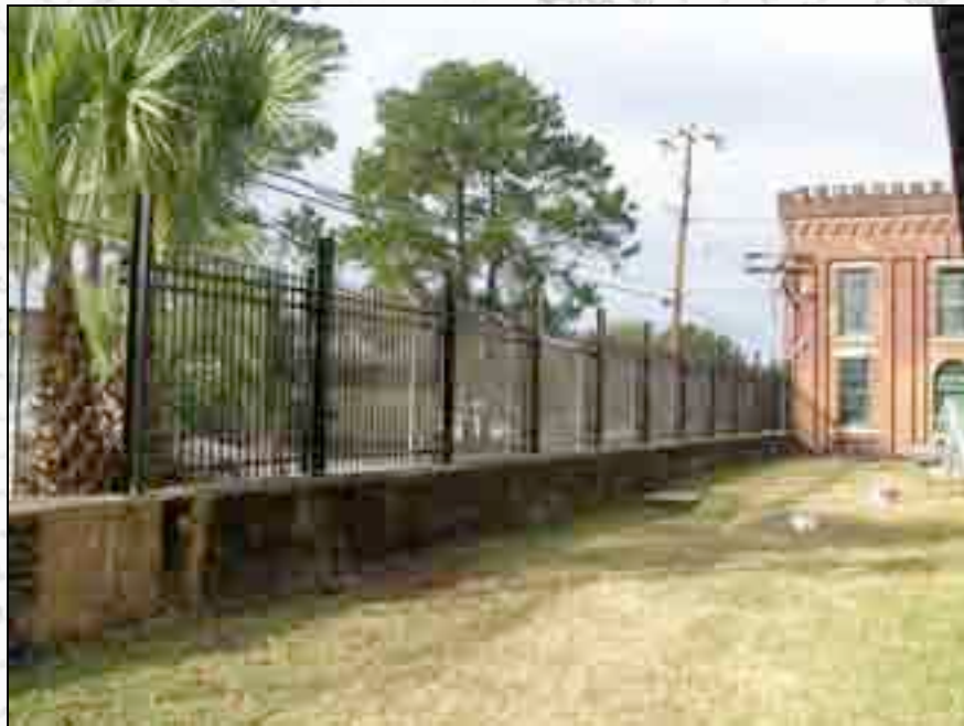
View looking west within the complex.
