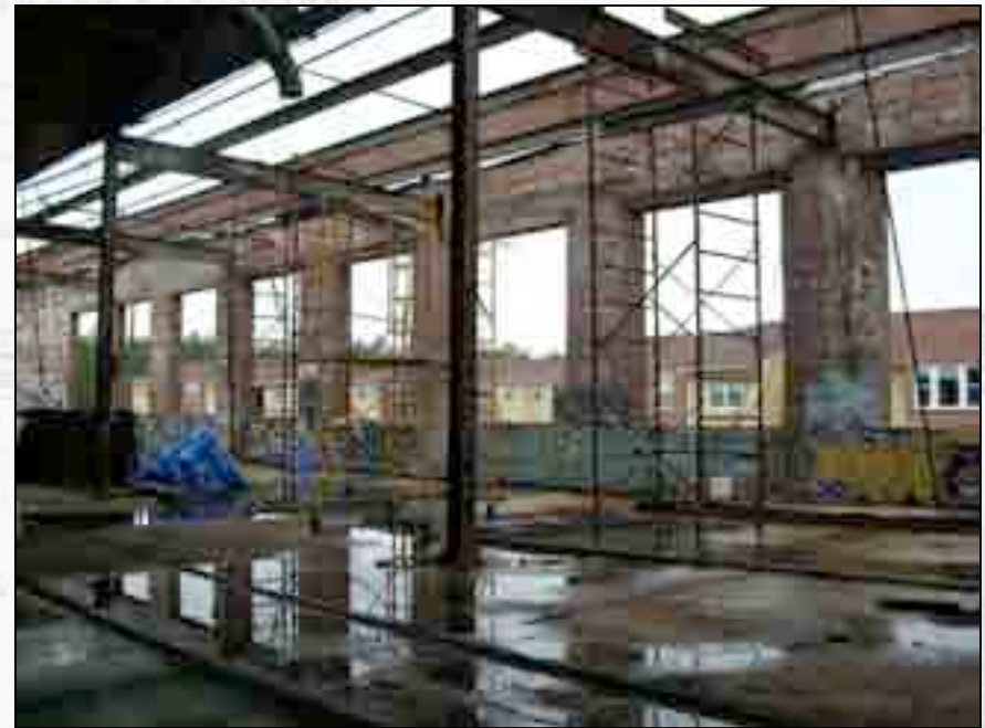
After windows were removed.
