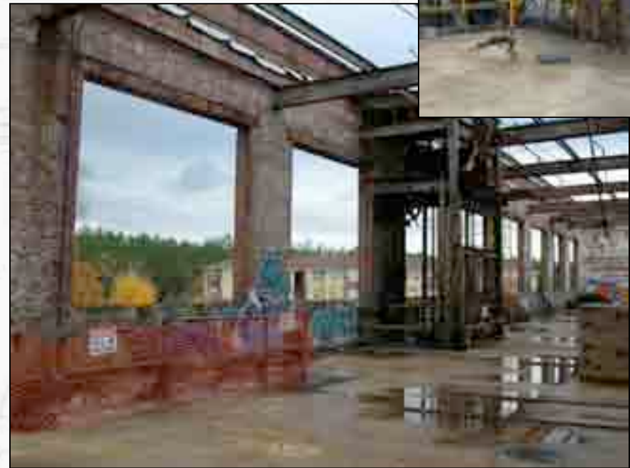
After windows were removed.
