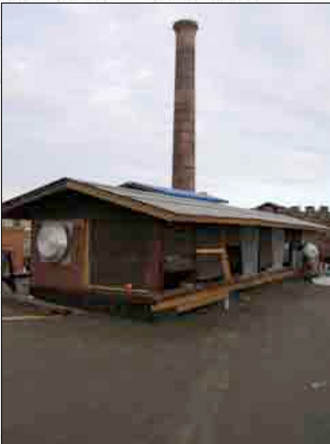
Monitor during restoration.
