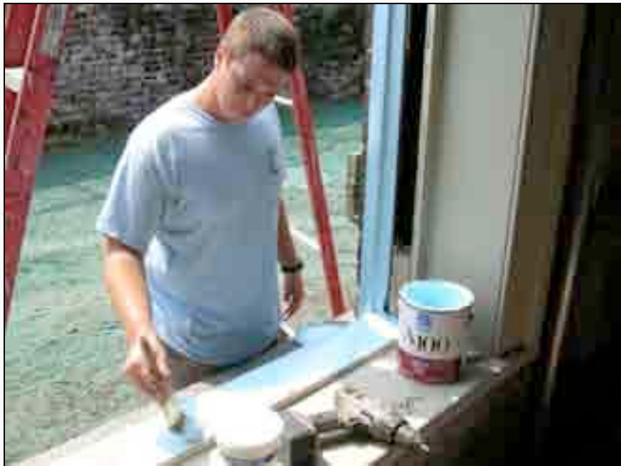
Ryan primes the window casing before the restored window is reinserted.
