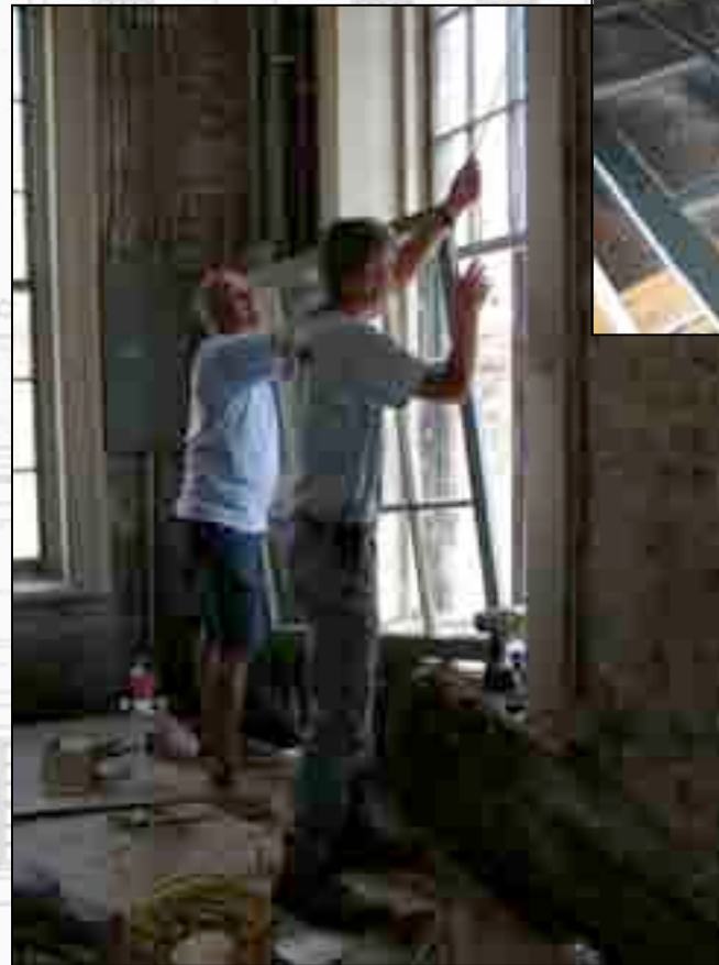
Kurt and Charles install a newly restored window.
