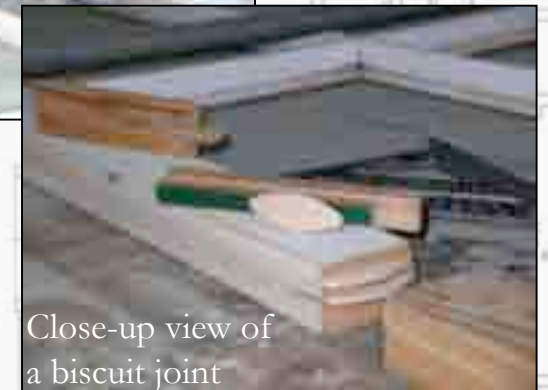
Don has removed the rotted bottom piece of a window from the Visitors Center and replaced it with new wood, joining the new pieces to the original frame with biscuit joints on the sides, and mortis and tenon joints at the corners.
