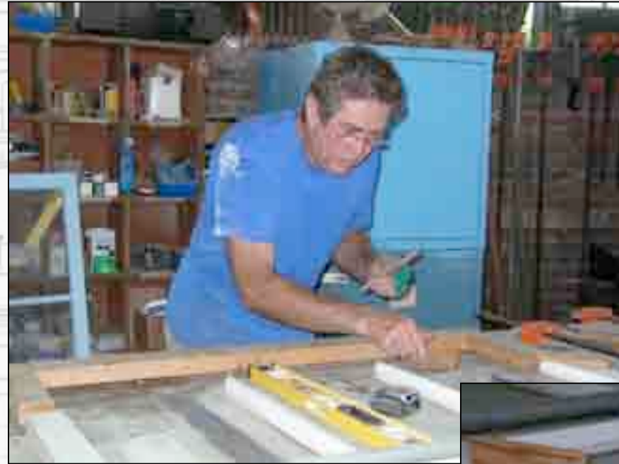
Don has removed the rotted bottom piece of a window from the Visitors Center and replaced it with new wood, joining the new pieces to the original frame with biscuit joints on the sides, and mortis and tenon joints at the corners.
