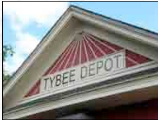
Close-up views of the freshly painted Tybee Depot.
