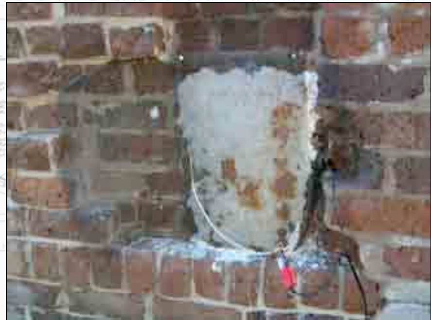
After 24 hours, the treated area is already showing signs of rust removal as oxygen is being transferred from the metal to the tissue through magnetic attraction.
