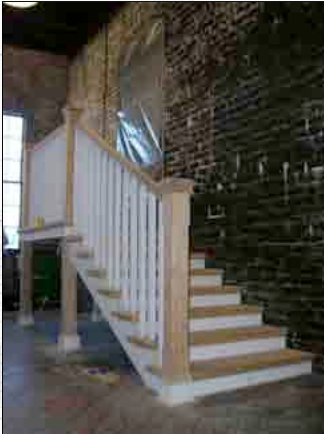
Stairs nearing completion.
