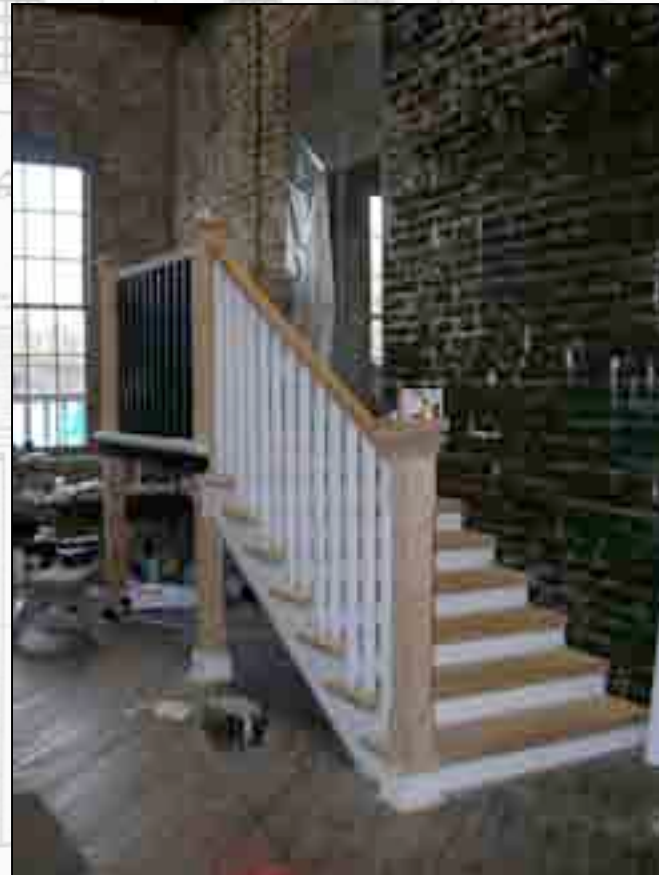
Paint is being applied to the new staircase.
