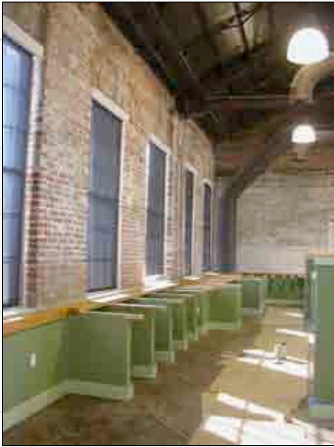
Interior wall with desk openings.
