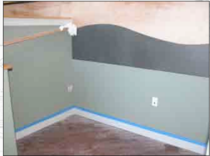
Cubicle before carpet and desk were installed.
