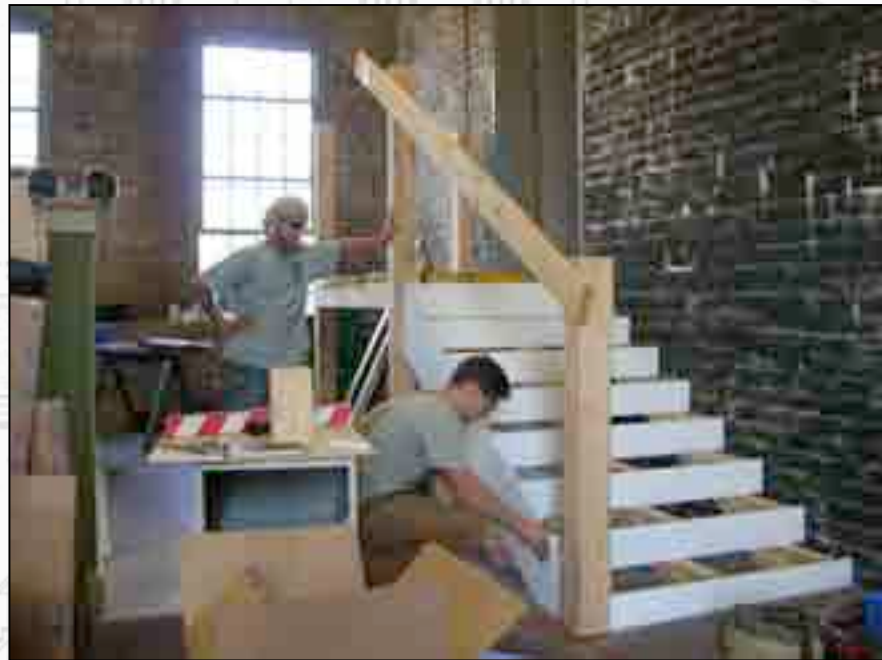
Ian and Nathan start constructing the stairs to the conference room.
