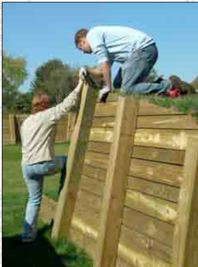
Amy and Joe measure the top portion of the post that needs to be cut.
