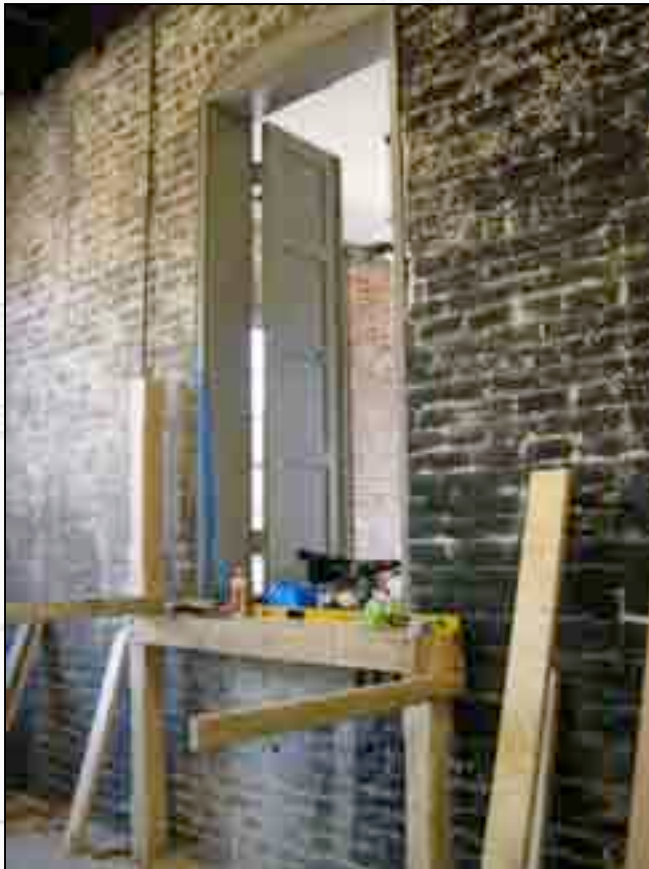
The frame for the new staircase is laid out.
