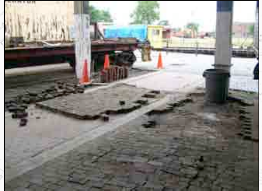
Present woodblocks are removed to make test patches before the full restoration process begins. Various mastics and sealers are being tested.
