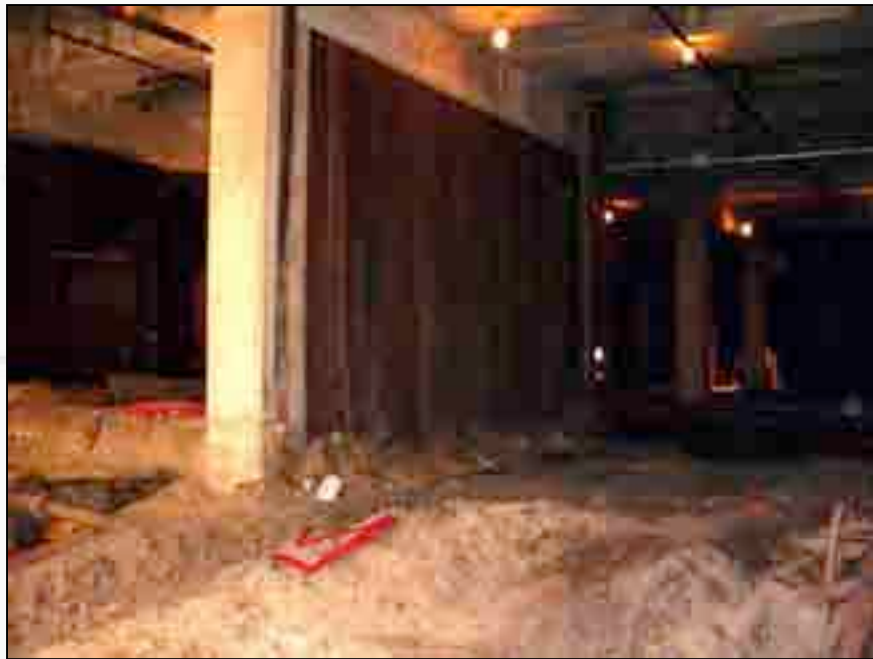
View of the wall before it was removed.
