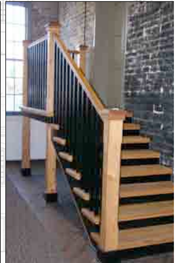
Stairway to the conference room was completed.
