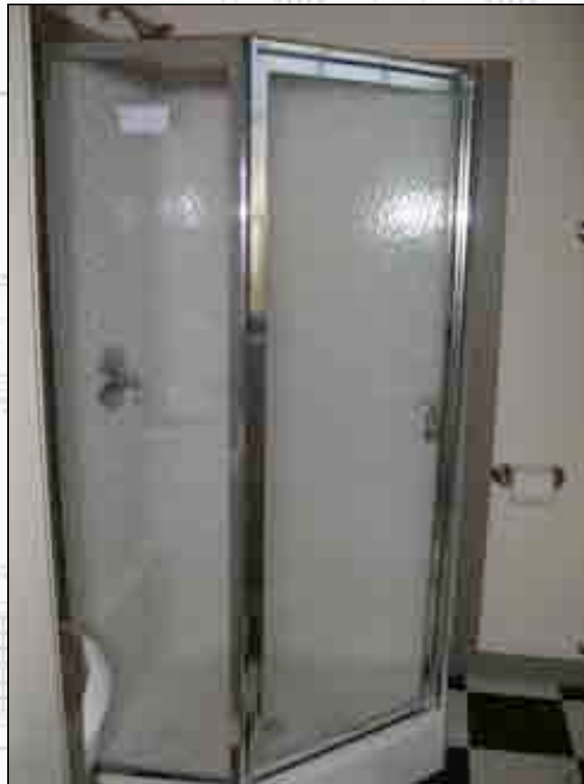
New shower was installed.
