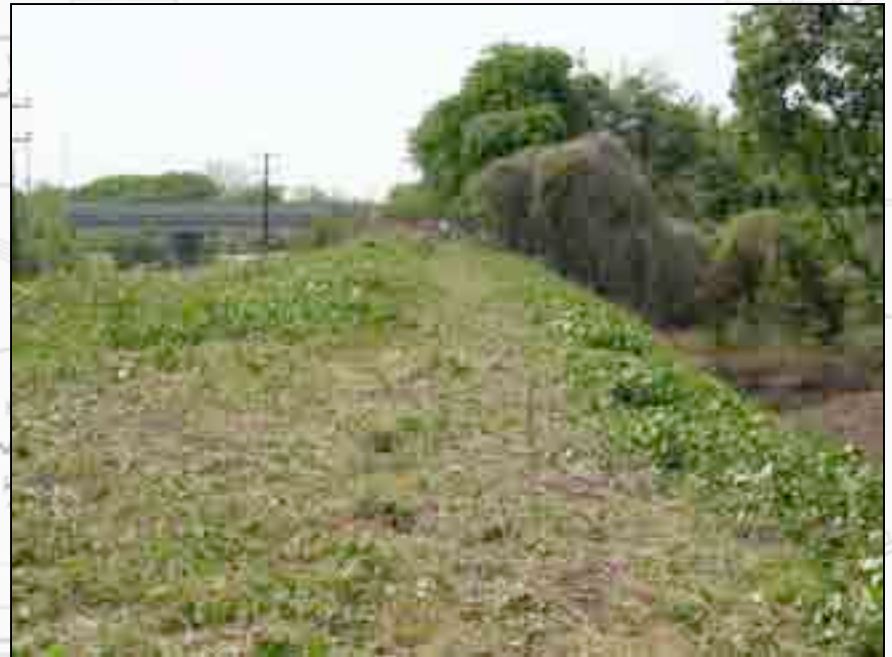
View from viaduct looking west towards I-16. The Preservation Team has cleared this area.
