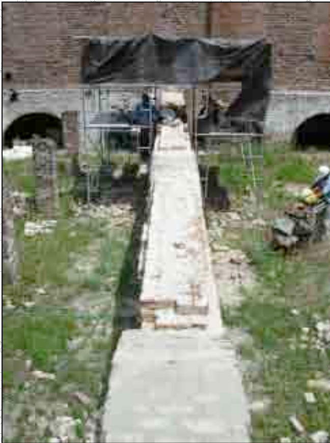
Top portion of foundation arches shortly after masonry restoration began.
