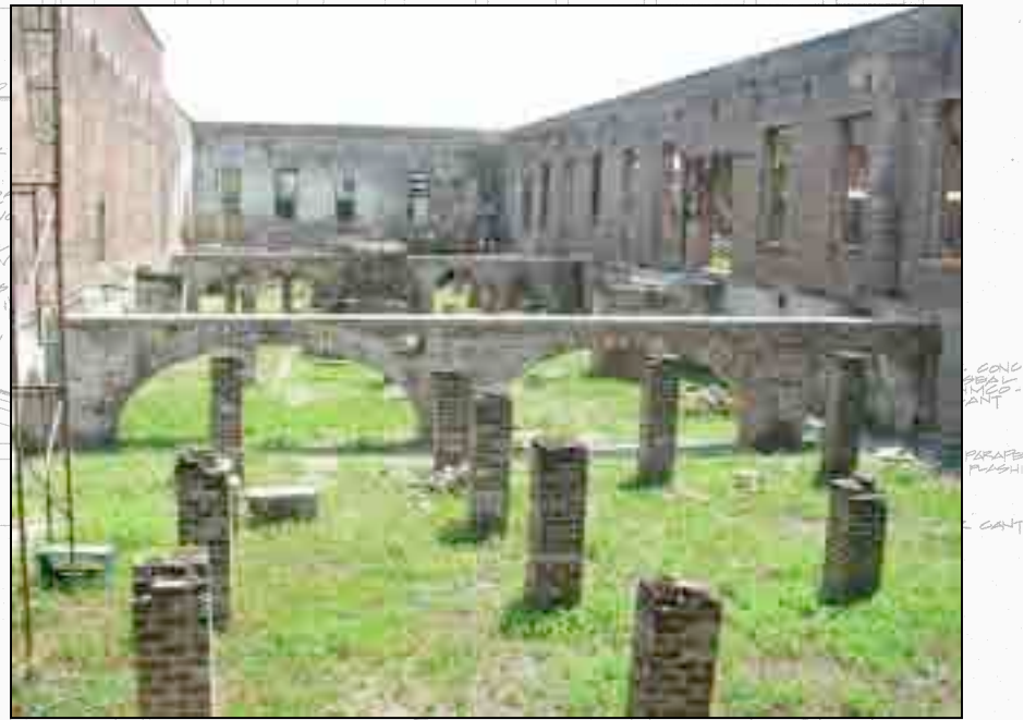
Current view of foundation arches that have been restored and rebuilt.
