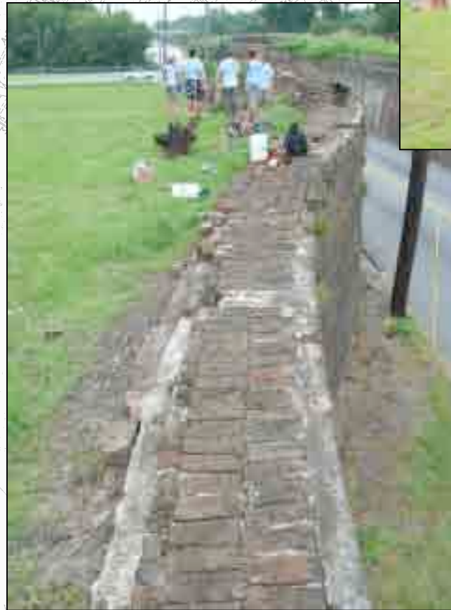
After all vegetation is removed, masonry repairs will follow.
