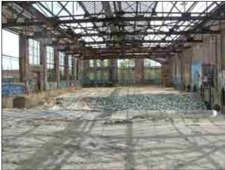
Interior of Coach Shop before windows were removed.
