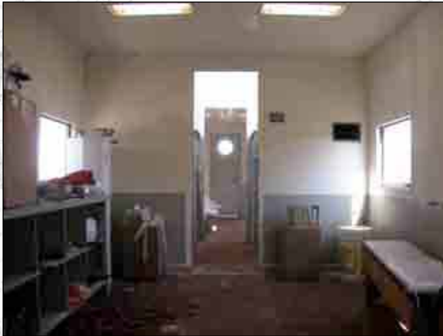
View of interior during construction
