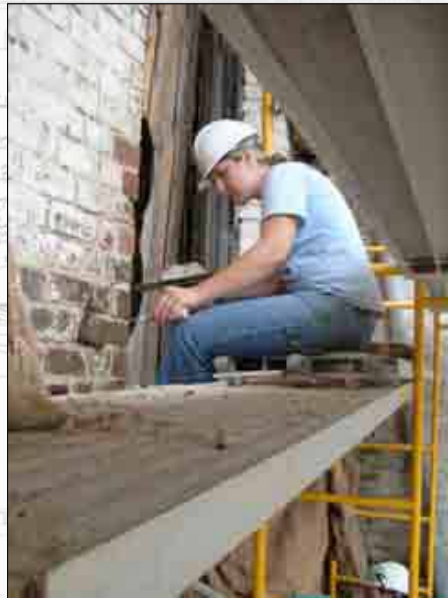
Tarin Erickson repoints a corner of a window opening.
