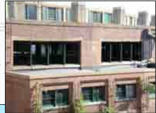
Close-up view after repairs
