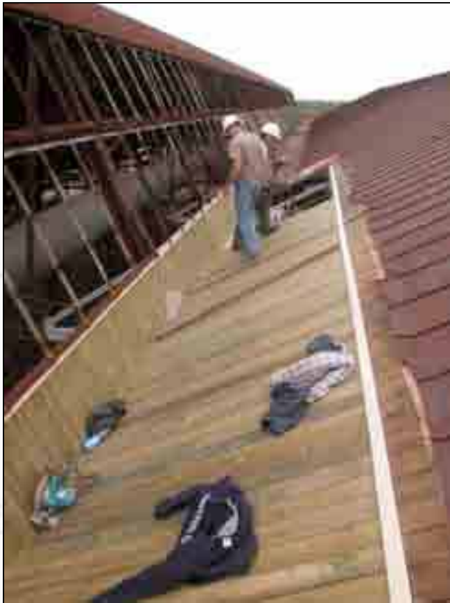
View from top of sawtooth roof.
