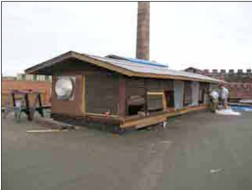
View of monitor shortly after restoration began.
