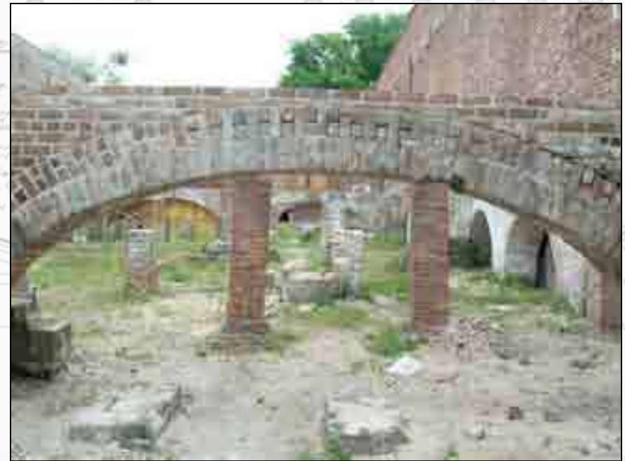
Current view of arch after masonry repairs.
