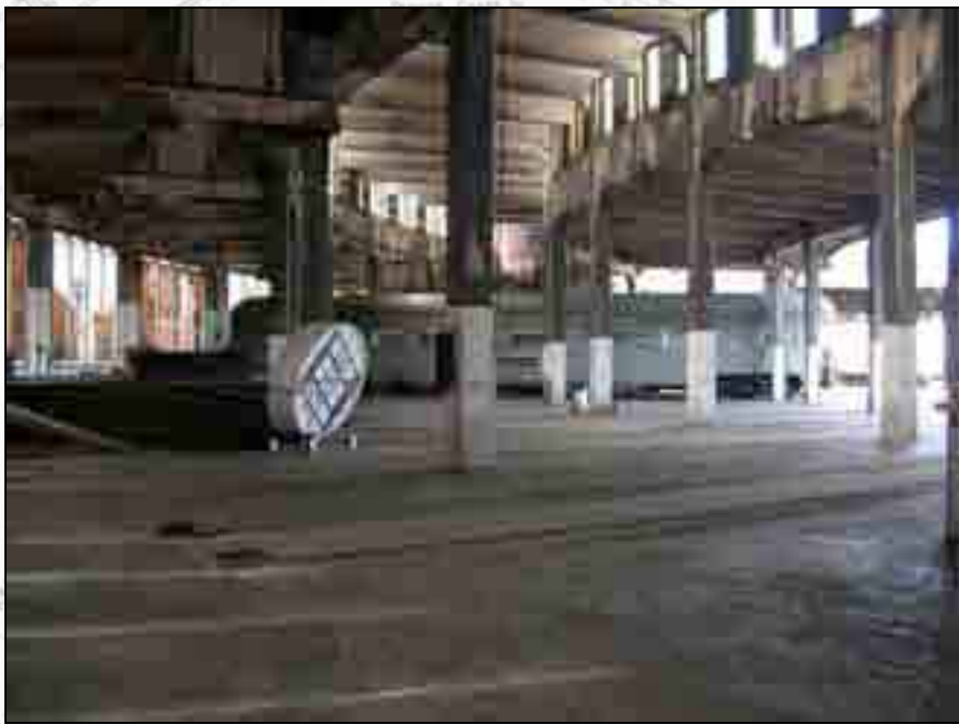
Overall view of restored wood block floors inside the Overnight Shed.
