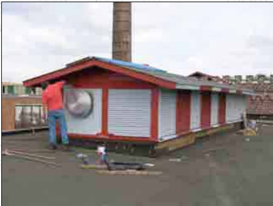
Kevin MacMillan applies the first coat of paint.
