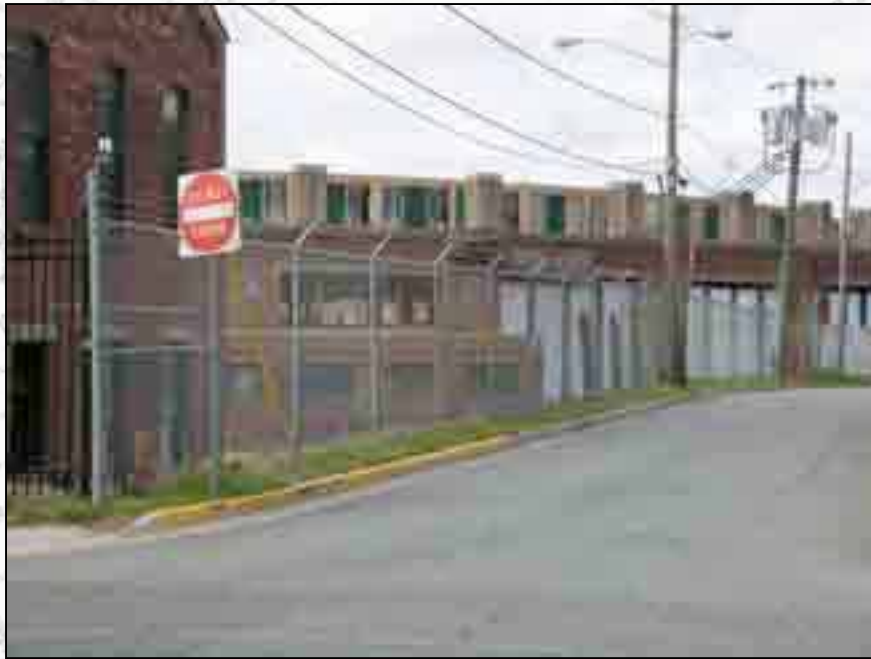
Chain-link fence at Purse Street
