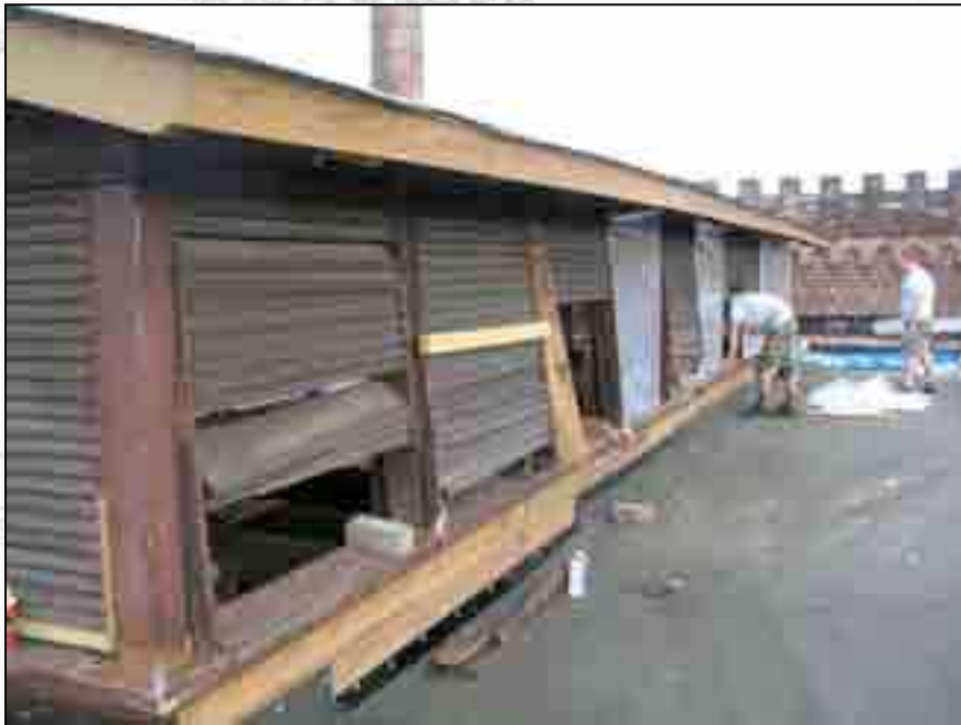
Another close-up view of monitor shortly after restoration began.
