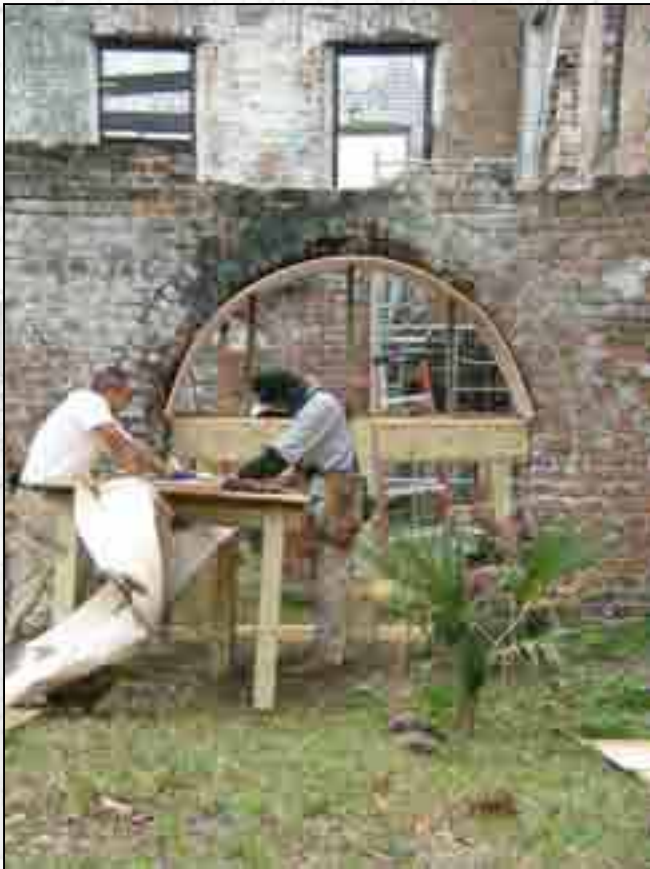
View of arch before masonry repairs.
