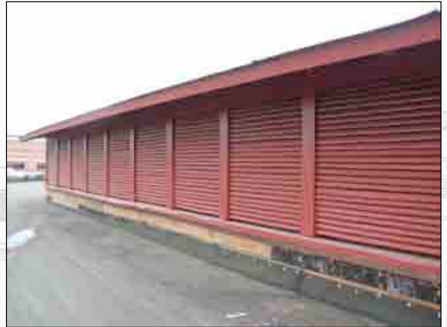
Deteriorated wood was repaired or replaced.
