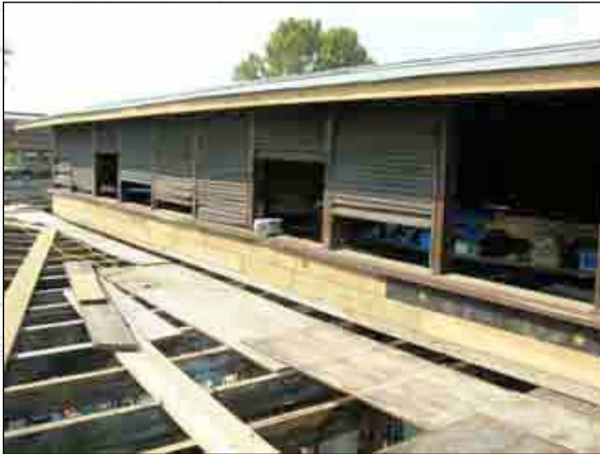
Close-up view of monitor shortly after restoration began.
