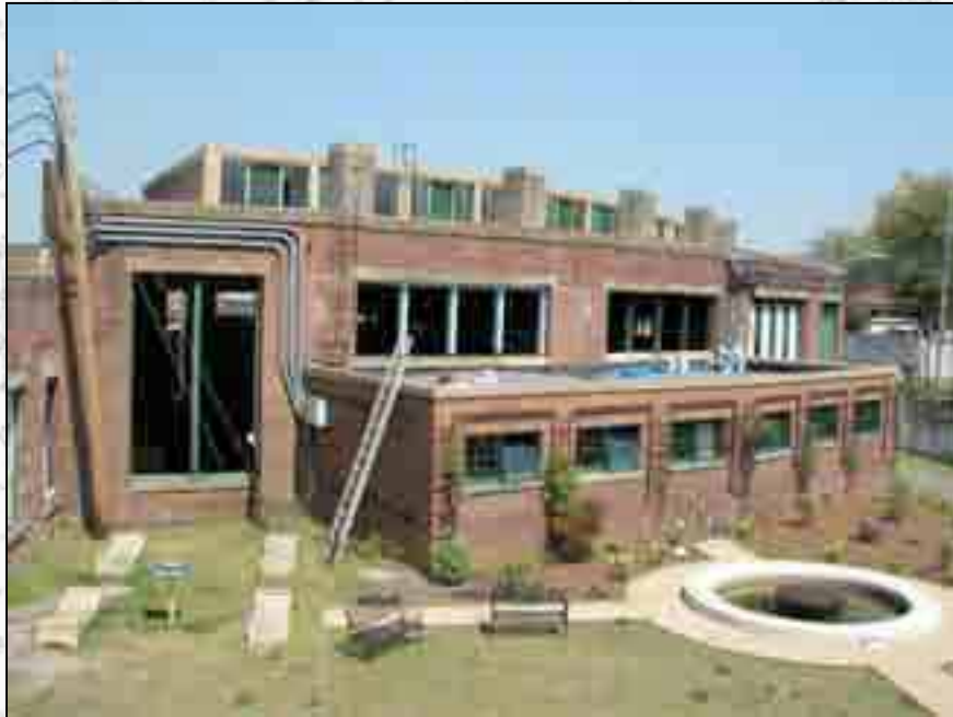
View during repairs
