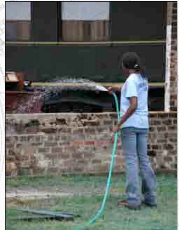
Mya Passmore rinses hydroseed away from the walls and foundation.
