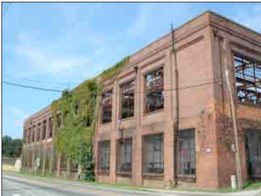
Exterior West Wall
