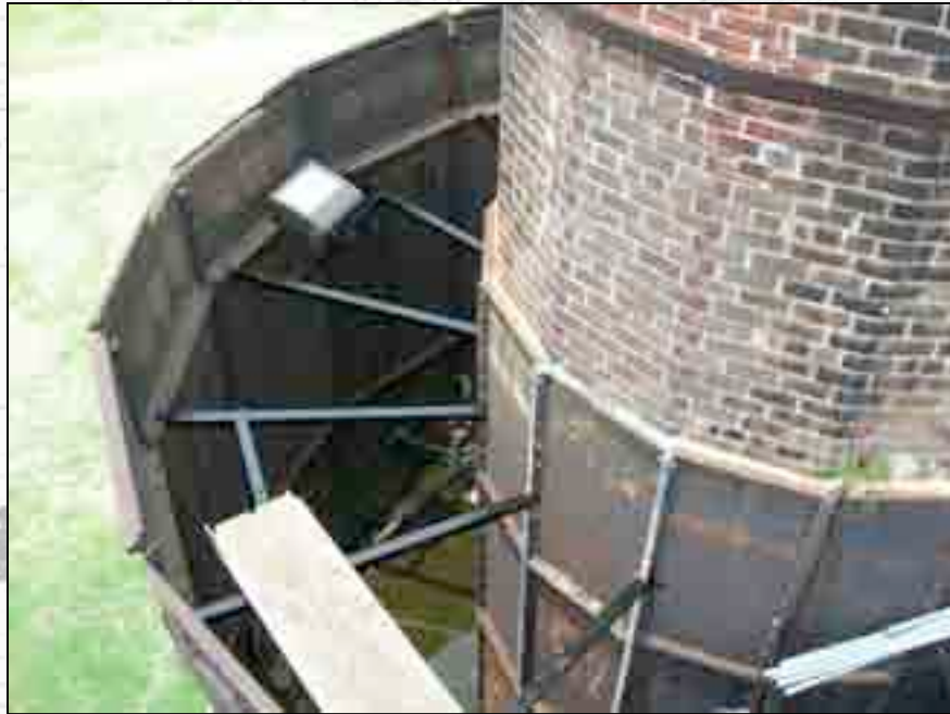
Repairs to Upper Circular Crack
