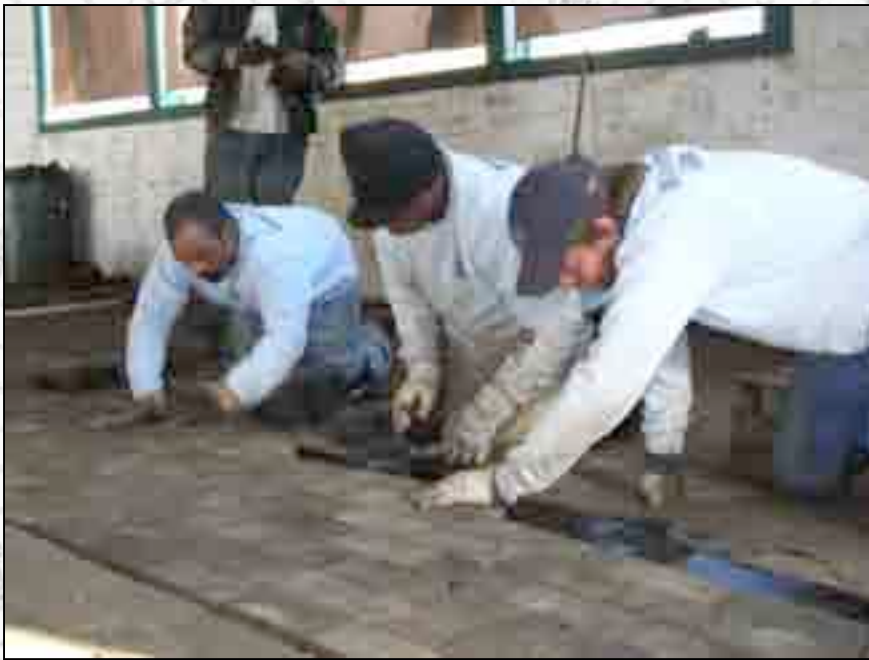
John Passmore, James Jackson, and Kevin MacMillan lay wood blocks at the rear wall of the Overnight Shed.
