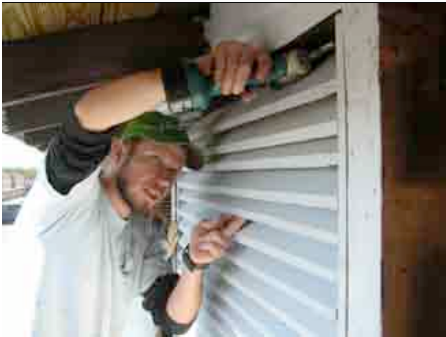
Nathan Harris secures the restored louvers into place.
