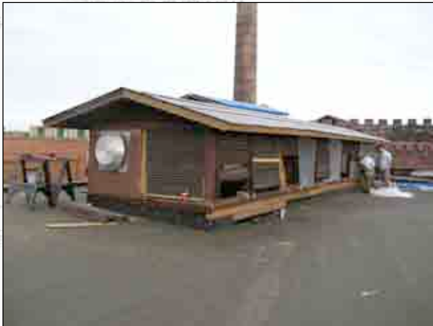
View of the monitor shortly after restoration began.
