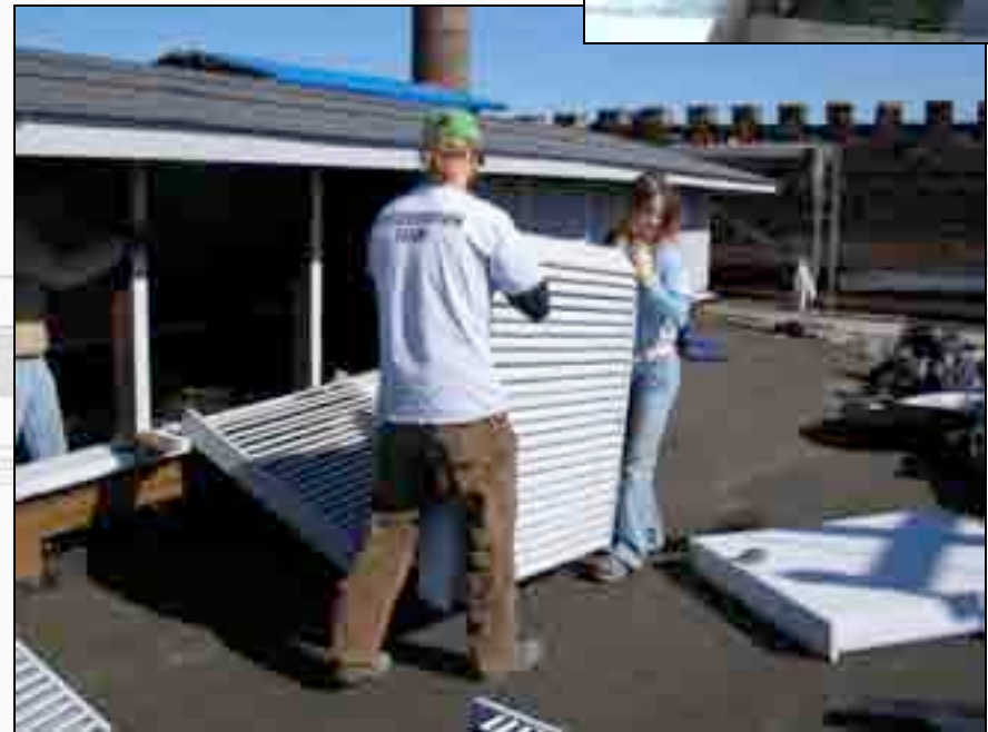
Nathan Harris and Amanda Smaridge position a restored louver frame into the monitor.
