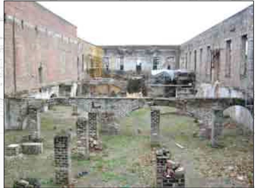
Current view of foundation arches that have been reinforced.
