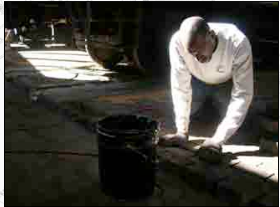
Anthony Temple finishes one of the last wood block lanes to be restored.
