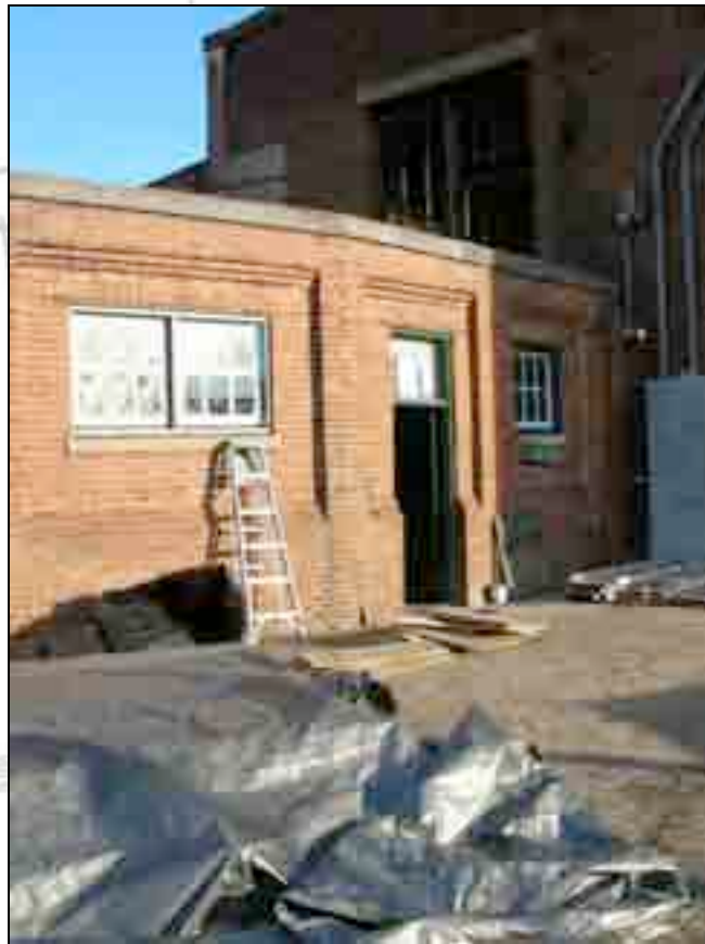
Close-up view of recently installed windows.
