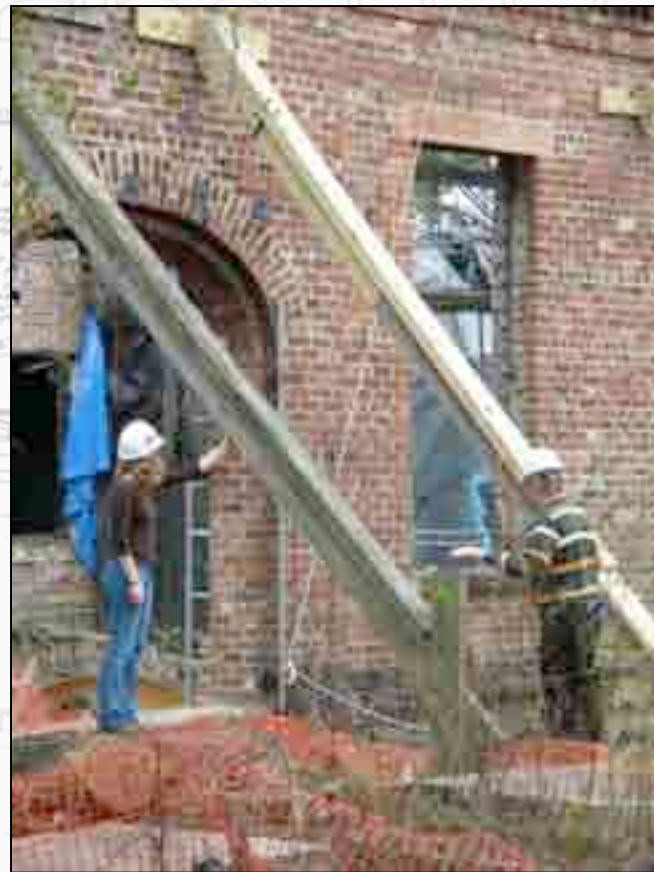
Becki and Hunter analyze recent improvements to the older bracing.
