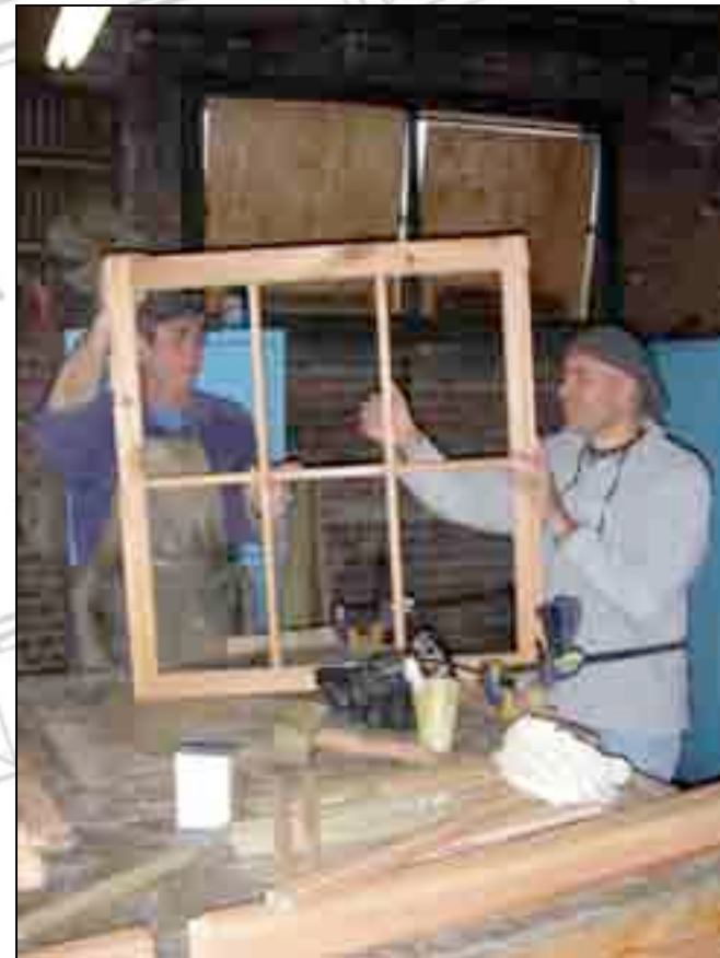
Carpentry Foreman Kurt Benton and Don Miller put finishing touches on one of the windows.
