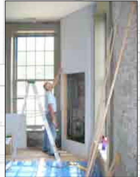
Kurt Benton builds a utility chase for the electric panels.
