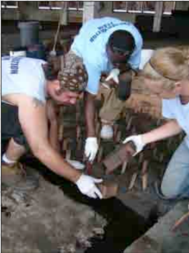
Preservation Team member, James Jackson, inserts shims while Bill Hersch and Amy Ver Beek lay woodblocks.
