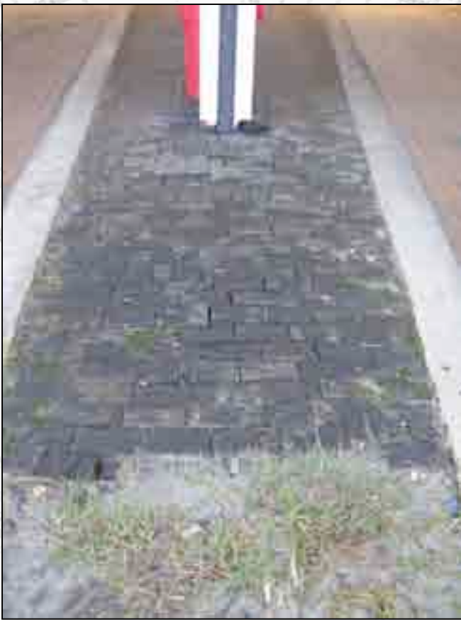
View of woodblock lane awaiting restoration.
