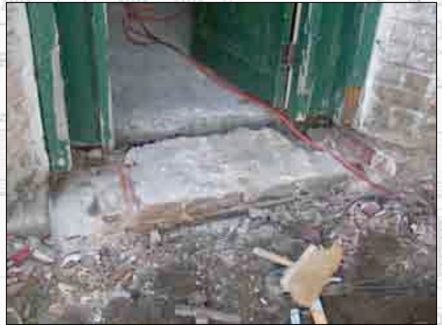
View of masonry found under rotted wood.
