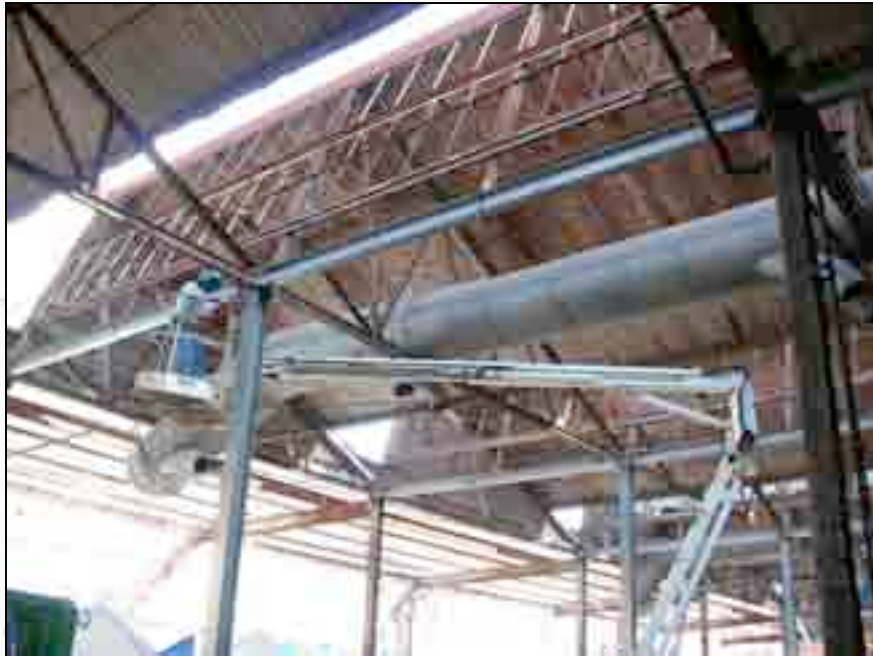
Bryan Law installs a cap plate to support cross beams.
