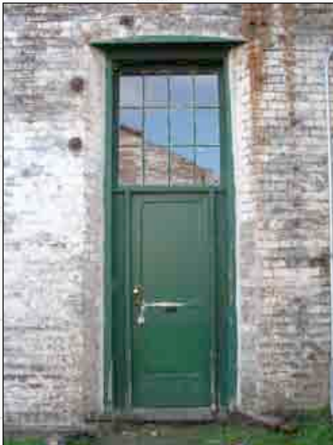
View of temporary door that was not original to the building.
