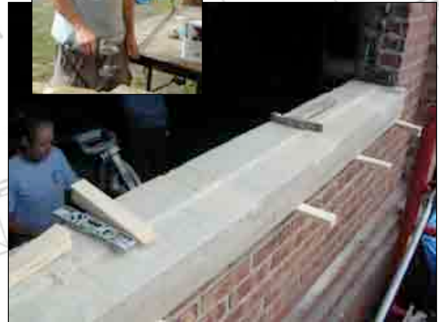
View of replacement sill.
