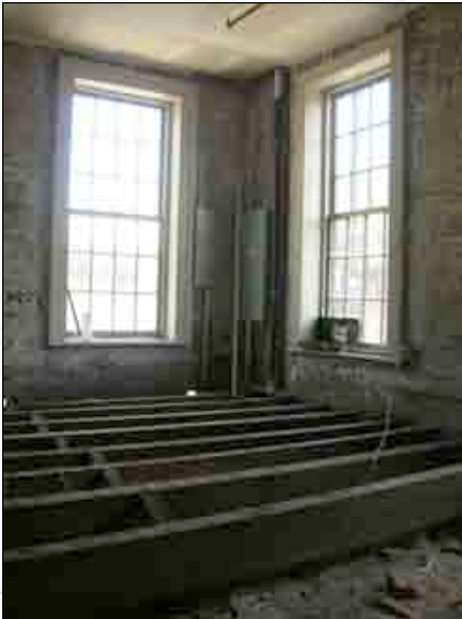
View of southeast corner of the room shortly after project began
