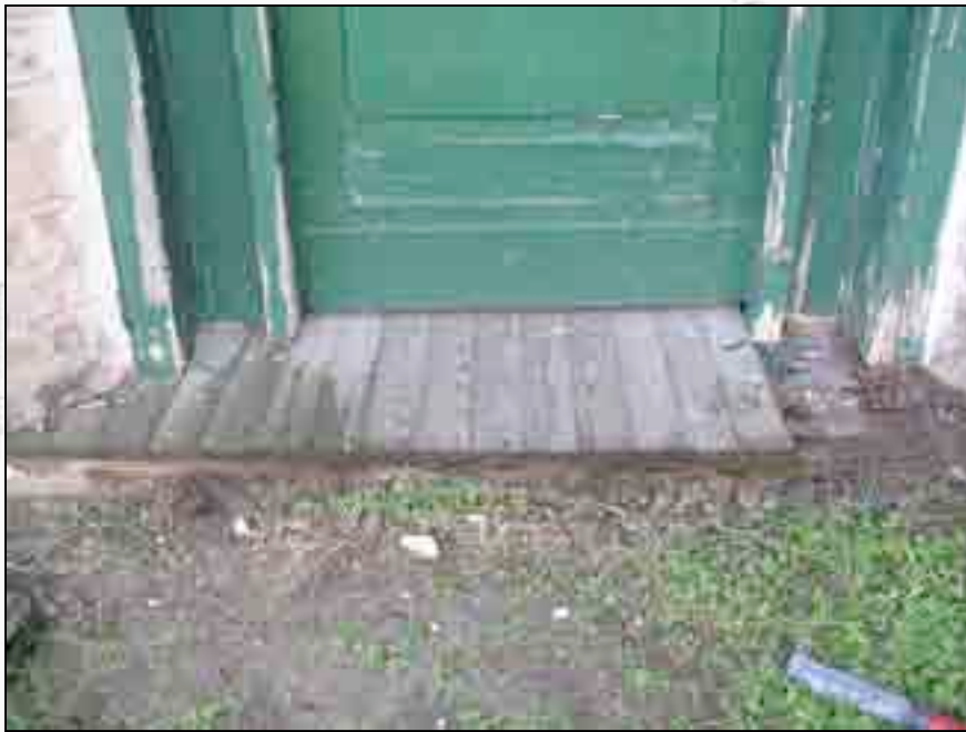
View of threshold before work began.
