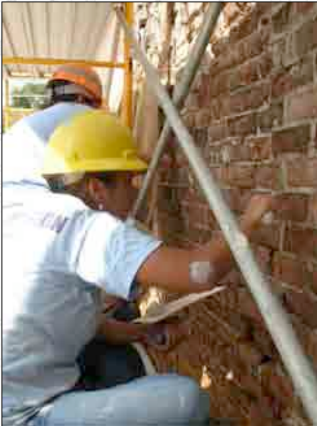
Ivey Ortiz repoints a section of the east wall.
