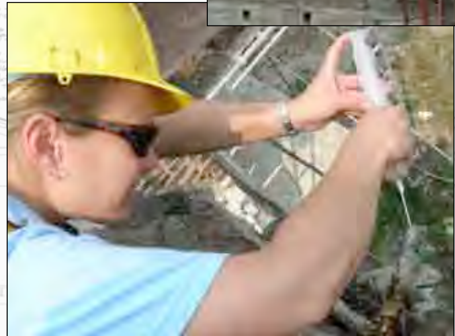
Then she injects the stem with an herbicidal solution that will kill the plant without harming the building.
