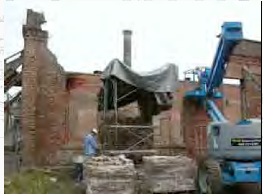
Rebuilding in progress.
