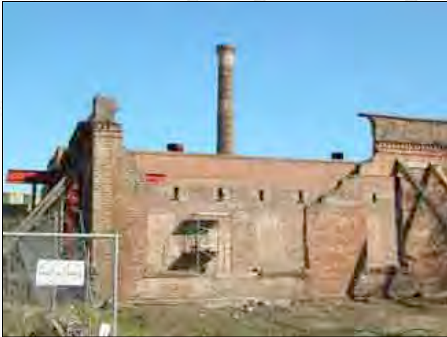
View of west wall before repairs.
