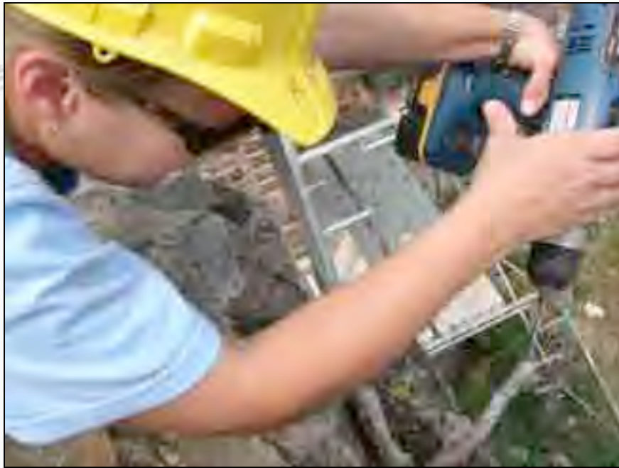
For large outcroppings of plant growth, Patricia drills holes into woody stems.
