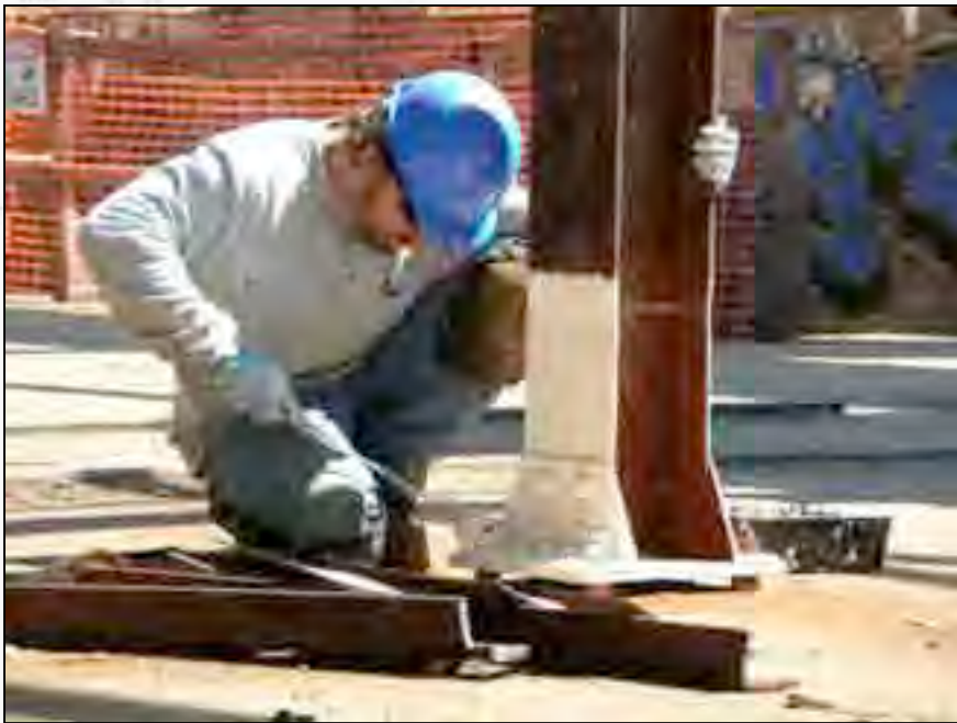
Kevin MacMillan primes the base of the column before painting it Central of Georgia bottle green.
