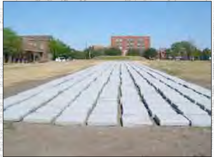
Current view of memorial walk. All 800 granite stones have been dry placed.
