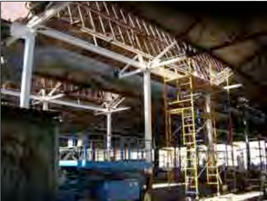
View of two northernmost sawtooth roof valleys shortly after project began.
